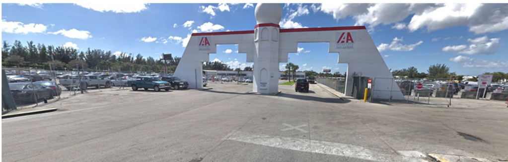
View of entrance of property highlighting Moorish Structure currently on site
