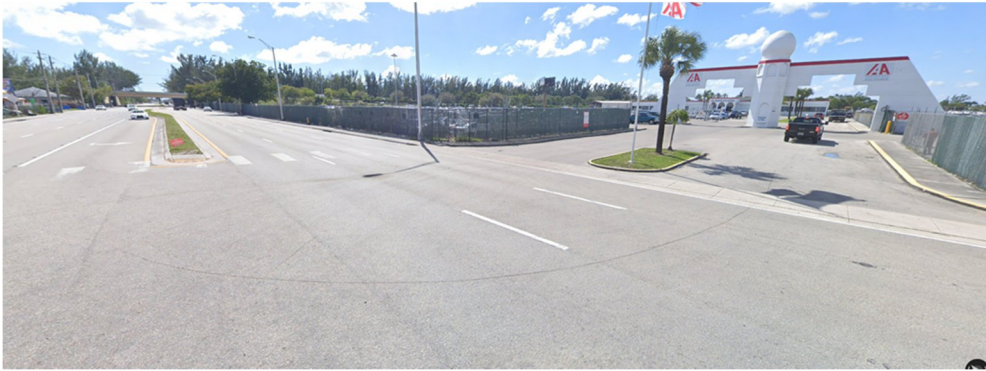
South View of property (South on Le Jeune Road facing State Road 924/Gratigny Parkway)
