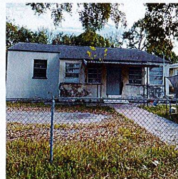
1330 Dunad Ave. - Deteriorated
