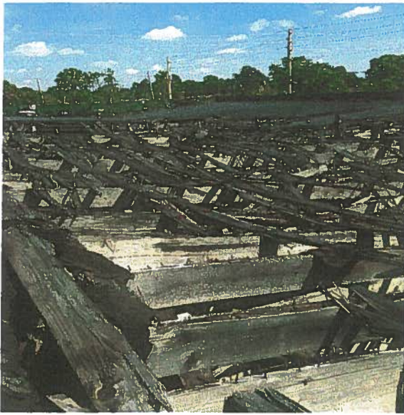
Overview of The Roof Framing
