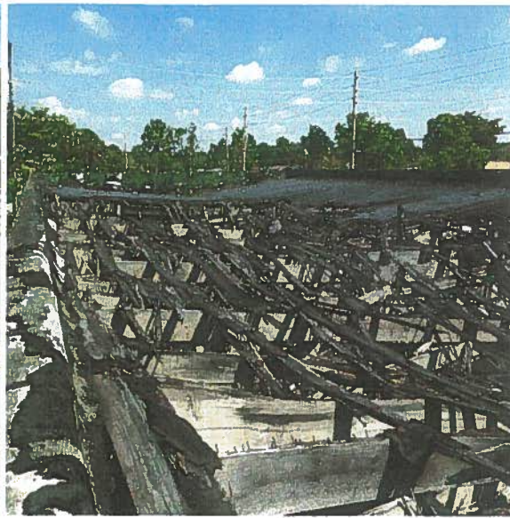
Overview of The Roof Framing
