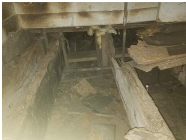
Replacing Damaged floor joists and roof rafters affected by termites
