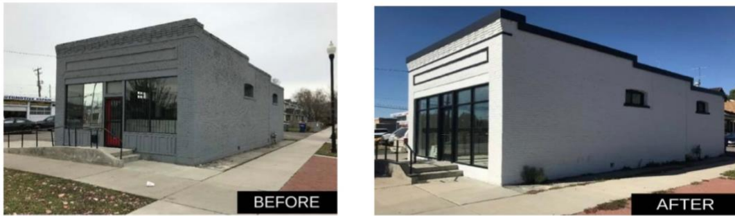
Figure XX: The revitalization of a neglected commercial district or residential neighborhood often begins with improvements to a single building or storefront. The before and after of a commercial building that participated in Salt Lake City's Facade Grant Program .
