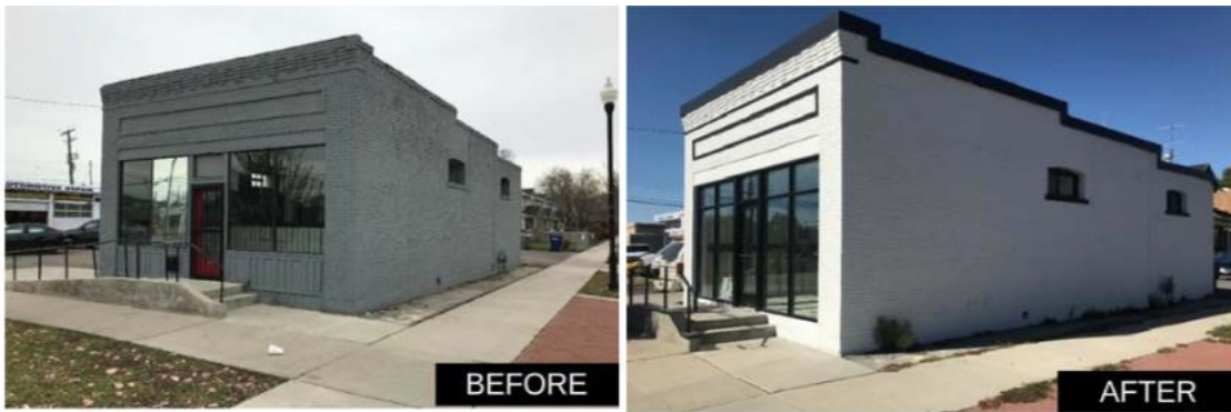
Figure XX: The revitalization of a neglected commercial district or residential neighborhood often begins with improvements to a single building or storefront. The before and after of a commercial building that participated in Salt Lake City's Facade Grant Program .
