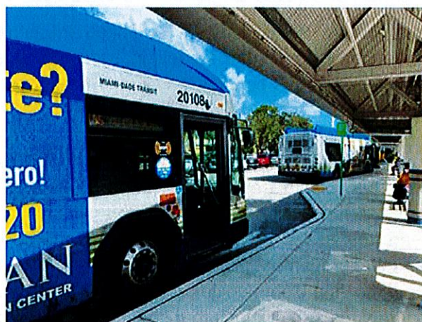
Figure 25: Opa-locka Tri-Rail Station Bus Bays
