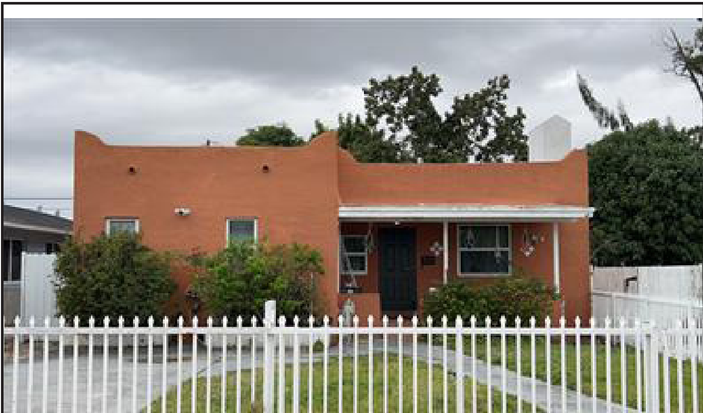
East Facade (Front facing Dunad Ave.) Photograph by Caleb Arsenault UF Historic Preservation Program Opa-locka Field Survey, Fla. Feb. 2023
