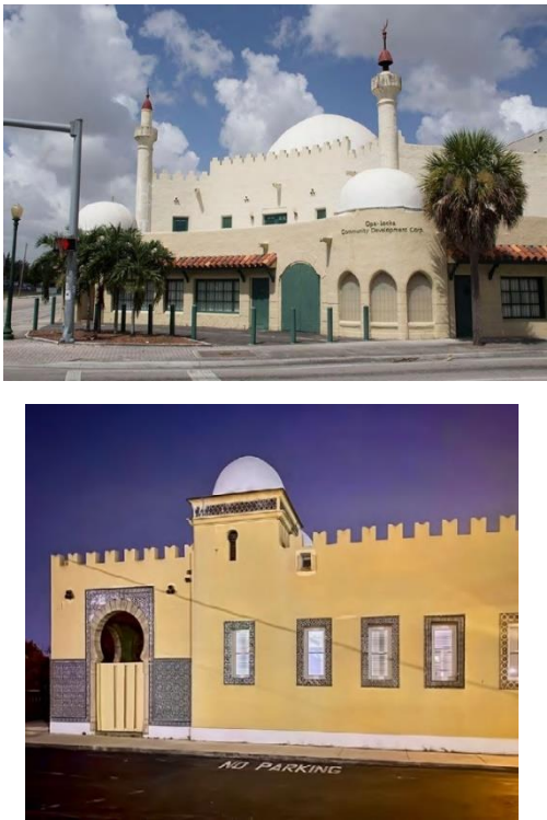
EXISTING OPA- LOCKA MOORISH ARCHITECTURE
