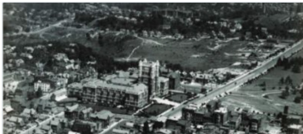
Construction begins on "District at Clifton Heights."
