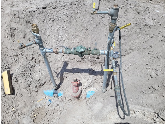
Photo No. 1 Prepared test location.
