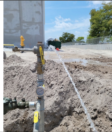
Photo No. 4 Released pressure to zero on all Water Line
