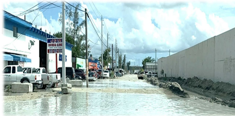
Existing Road Conditions
