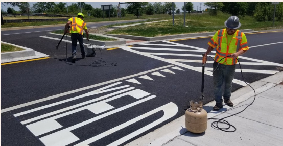
DeGemmill. "Roadway Construction Curb and Gutter Example." Photograph, 2023. https://www.degemmill.com/content/uploads/2023/03/20200603_131955.jpg .
