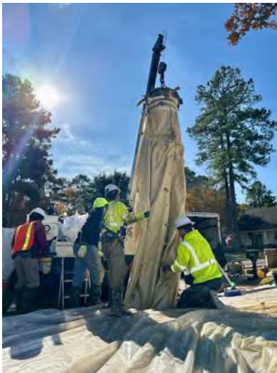
Liner Raised into Position
