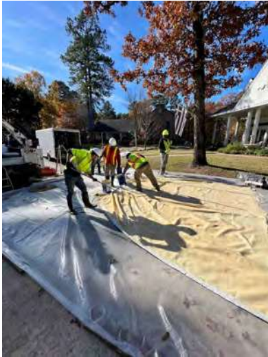
Liner Saturation w Epoxy
