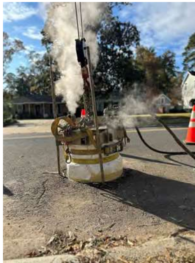
Curing w/ Air & Steam
