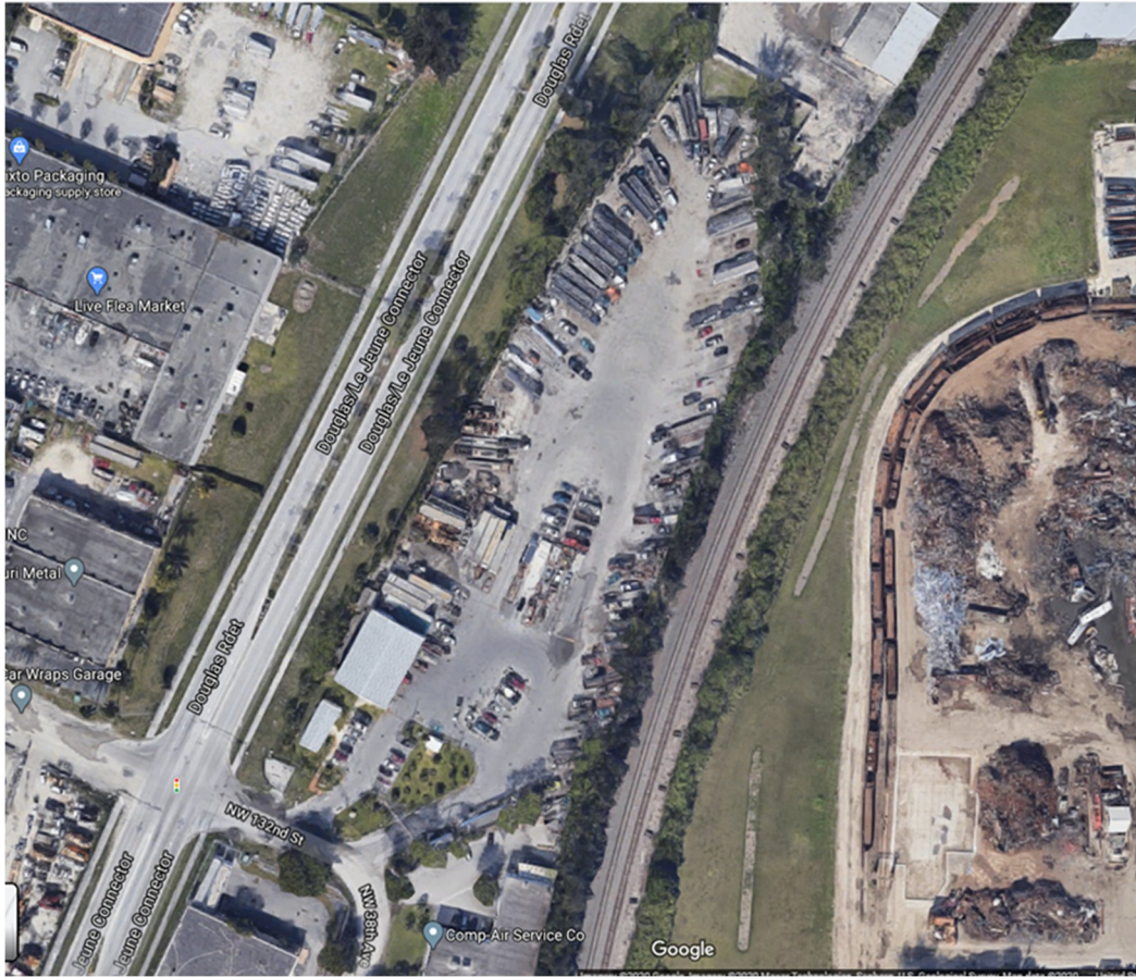
Enlarged Aerial View of 3805 NW 132 Street
