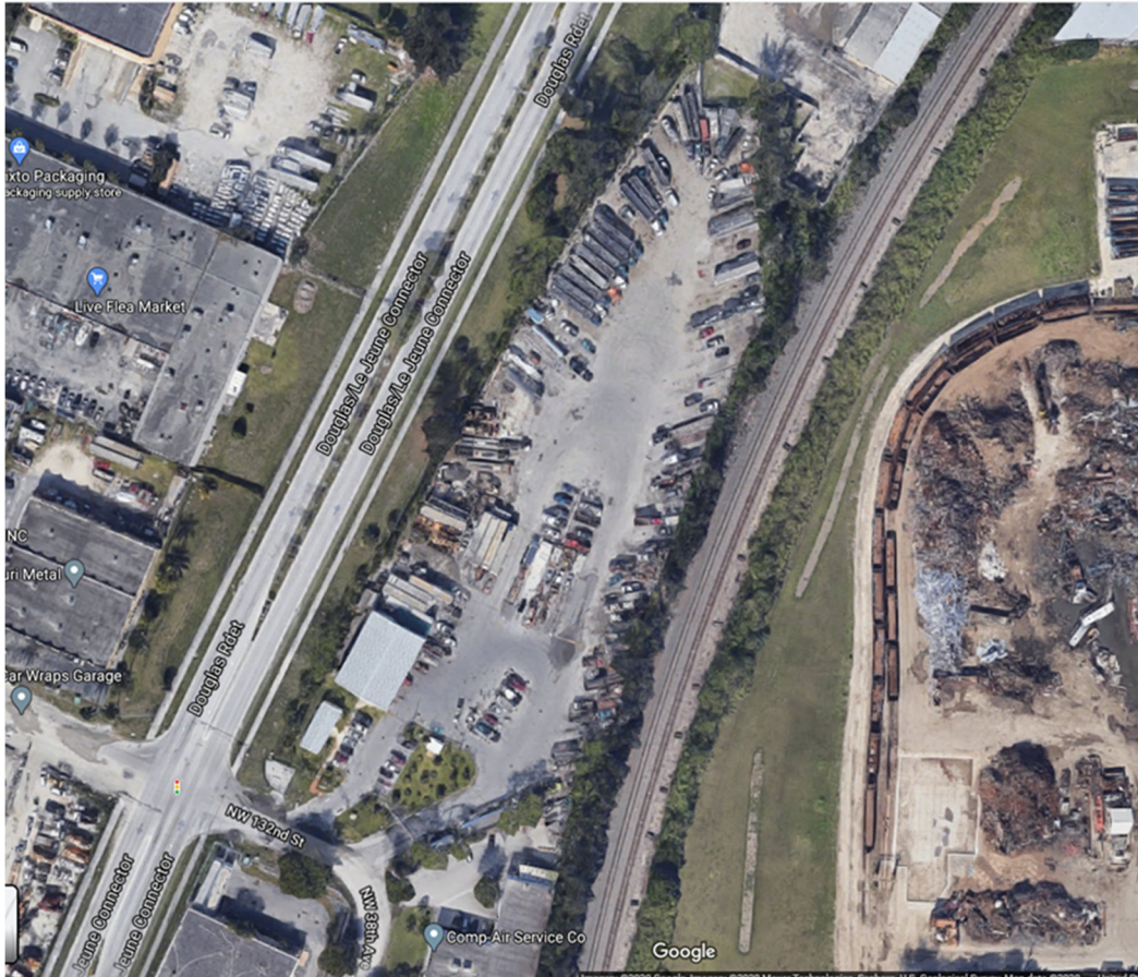
Enlarged Aerial View of 3805 NW 132 Street
